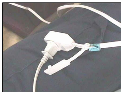
Electrical cords daisy-chained
