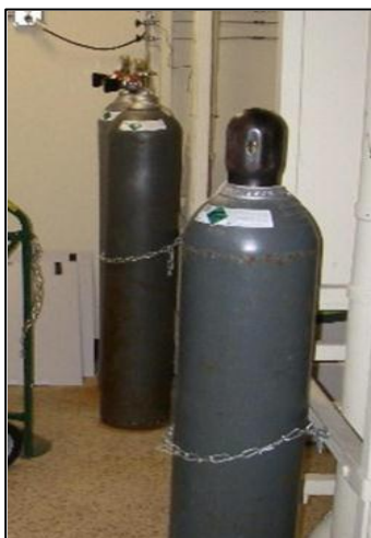
Acceptable method of securing a cylinder
